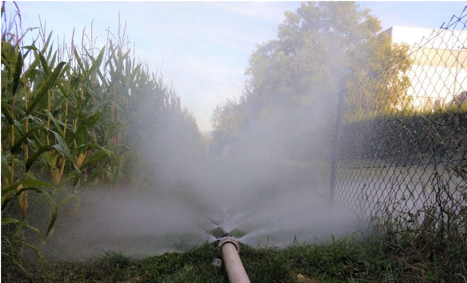
Figure 3 Functional test of the Boundary Cooling Device
